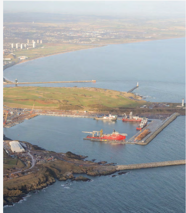
Amount invested: £35 million to create Scotland's largest port
