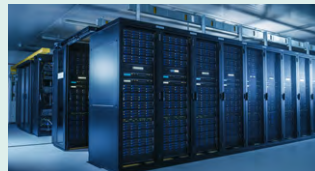
Data security and digital infrastructure
